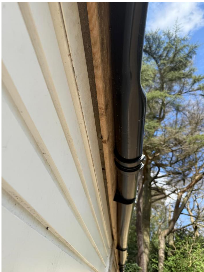
Figure 5. Evidence of sealed fascia
